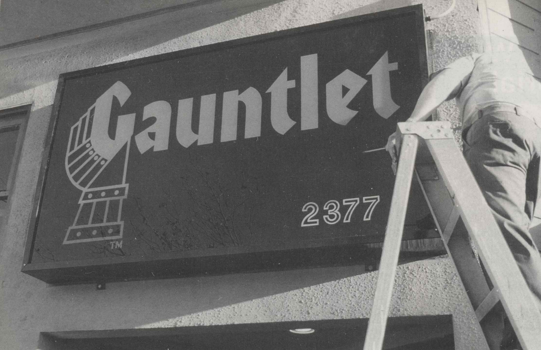
The illuminated sign over the front door is installed.*
